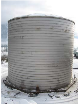
Water System Reservoir
