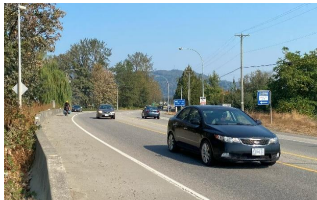
Figure 9: Existing MoTI Roadway
