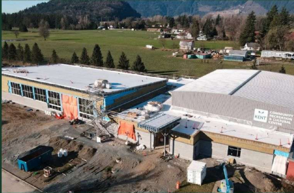
Lets'emó:t under construction, April 2026. (District of Kent)
