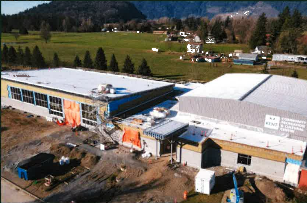
Lets'emó:t under construction, April 2026. (District of Kent)
