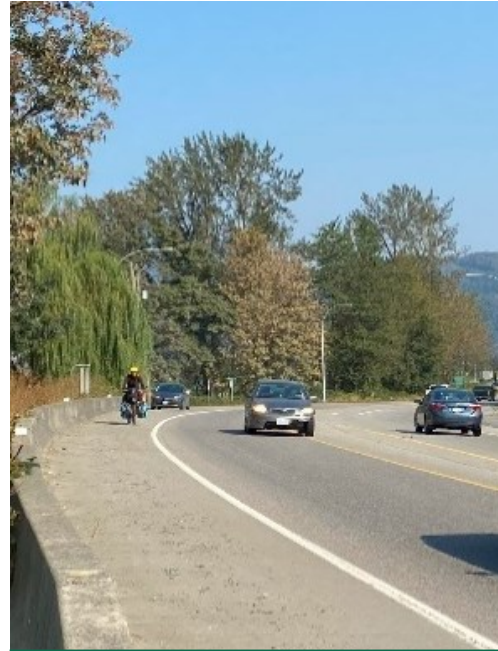
Upgrade Existing MoTI Facility
