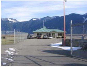
Waste Water Treatment Plant
